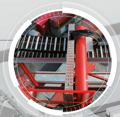
Rail Mounted Gantry [RMG]
